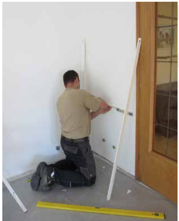
4 - Install the wall brackets
