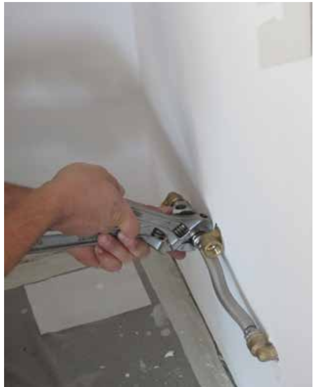
14 - Tighten firmly to ensure that they are leaktight
