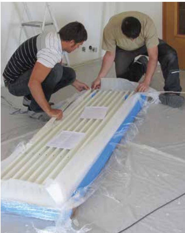
3 - Measure the centre-to-centre distance between the fixing brackets on the radiator. Caution: check the dimensions (1) very carefully
