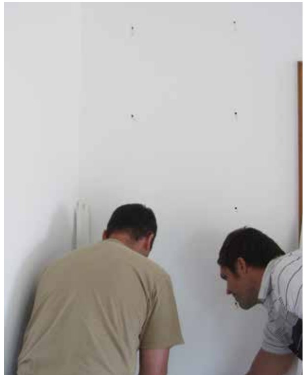
6 - Drill holes ready to take brackets with screws and rawl plugs suitable for the wall. Hang the brackets on the supporting wall.
