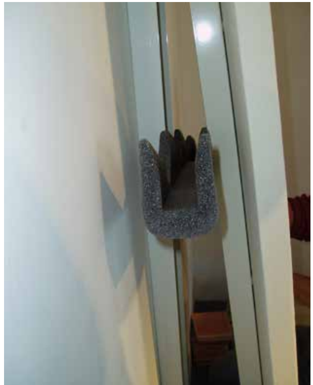
21 - Once the radiator is fixed at the top, insert a spacer to hold the radiator away from the wall
