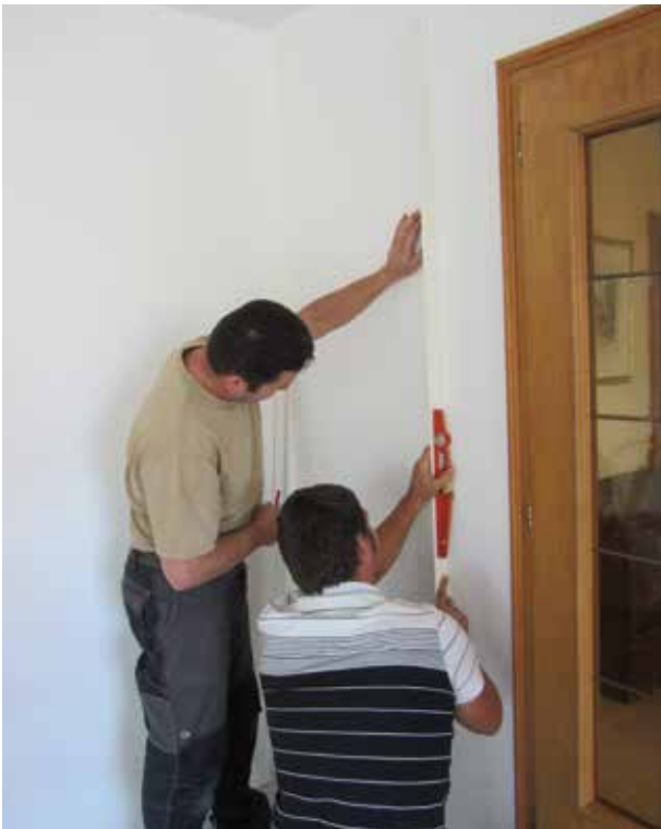
5 - Check that they are straight using a spirit level
