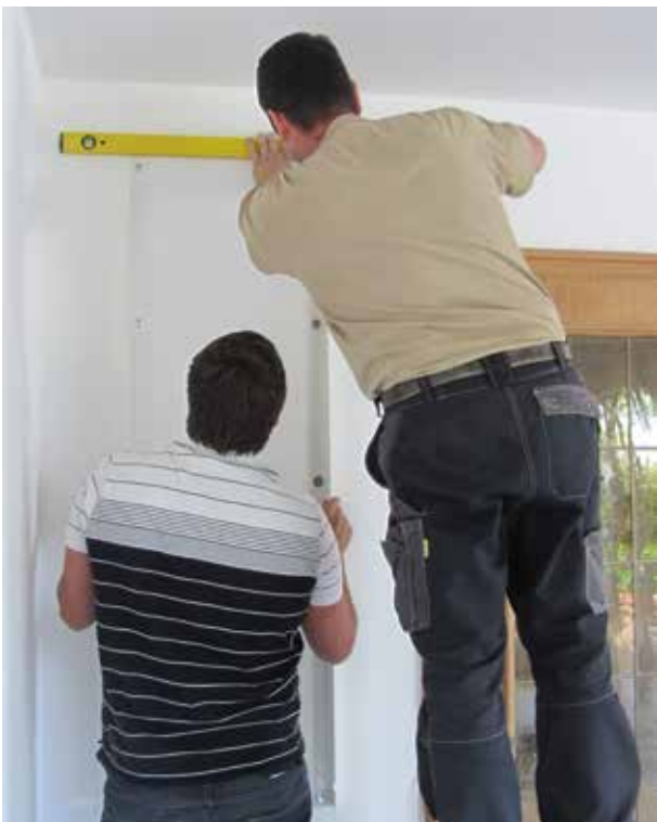
7 - Fit the brackets and use a level across the top to check they are straight
