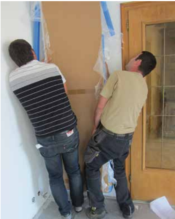
20 - Use two people to lift the radiator with the radiator lifting tool and attach the radiator to its brackets
