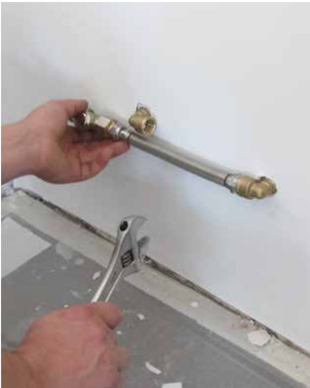
13 - Connect the hoses and valves to the wall connections
