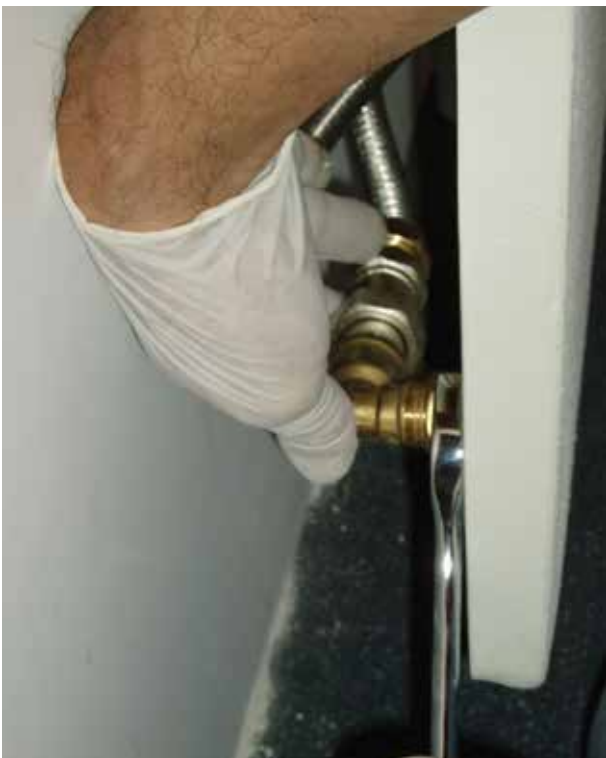
22 - Put on the gloves provided then connect the valves to the radiator.
