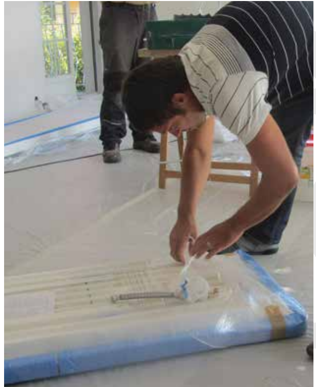
2 - Undo the protective plastic wrapping, but only on the back of the radiator, to release the brackets and connections
