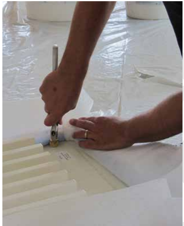
10 - Unscrew the plugs on the radiator
