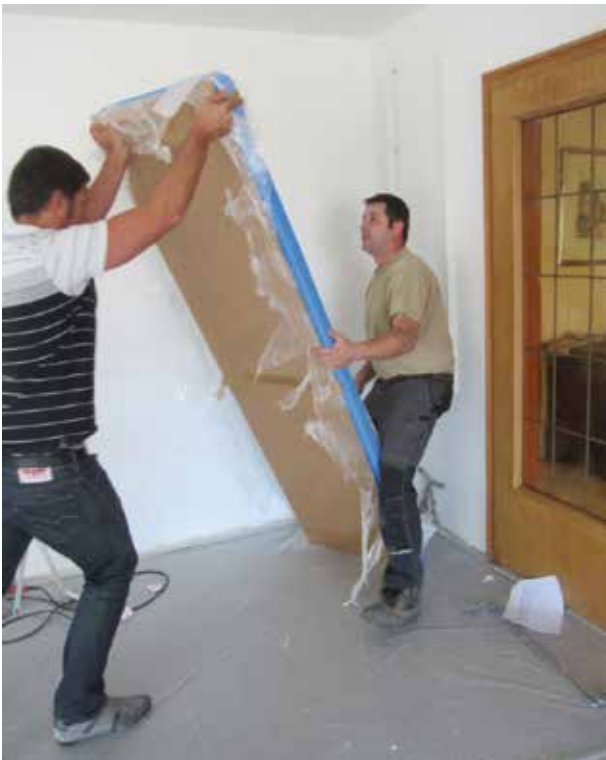
17 - Keep all the protective blue foam packaging in place
