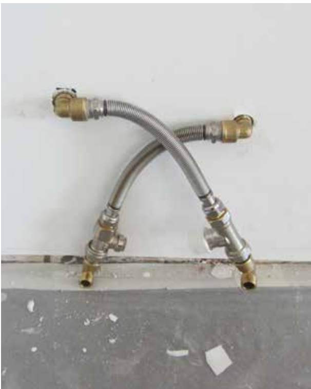
15 - Hoses and valves installed correctly
