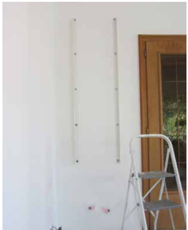
8 - Pipe apertures and brackets installed correctly
